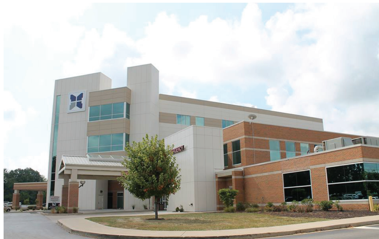
▲ Decatur County Memorial Hospital
